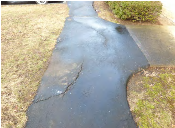
Typical asphalt walkway paving sub-base failure.
