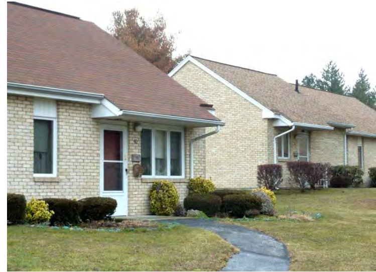
Newer asphalt roofing on building in the foreground and older asphalt roofing on the building behind.
