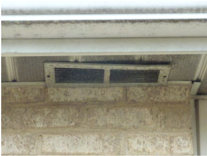
Typical grille condition at building soffits.
