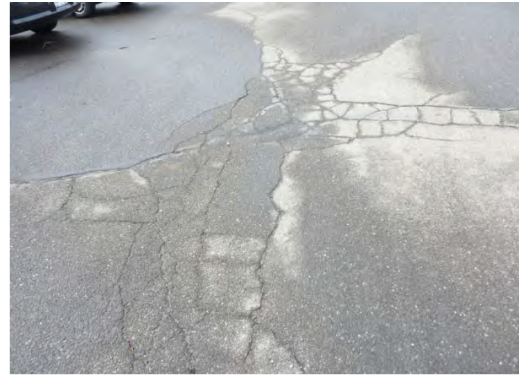
Typical asphalt drives paving sub-base failure.
